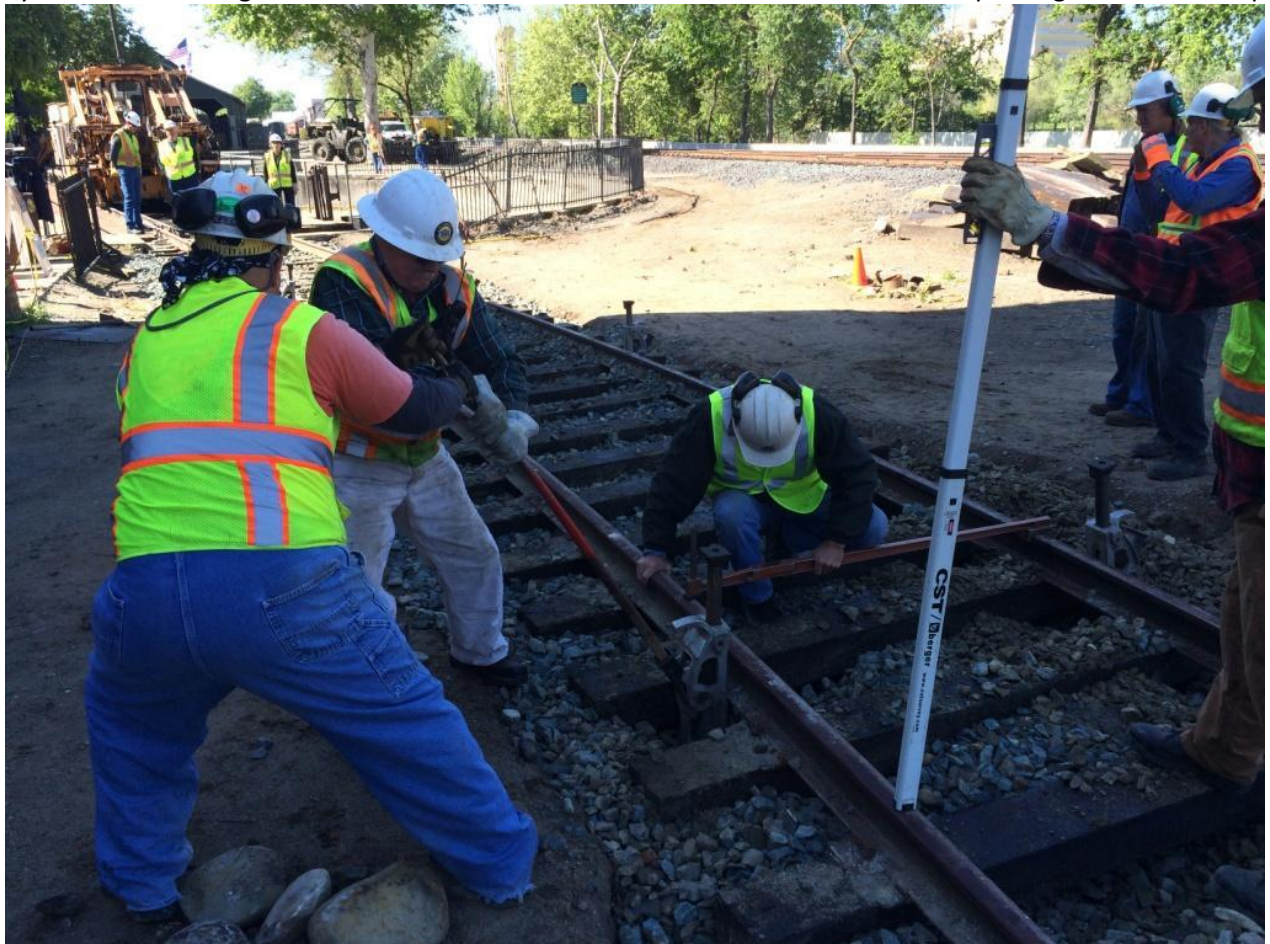
Mike F. and Mike H. struggle to jack the track as Alan measures track level
