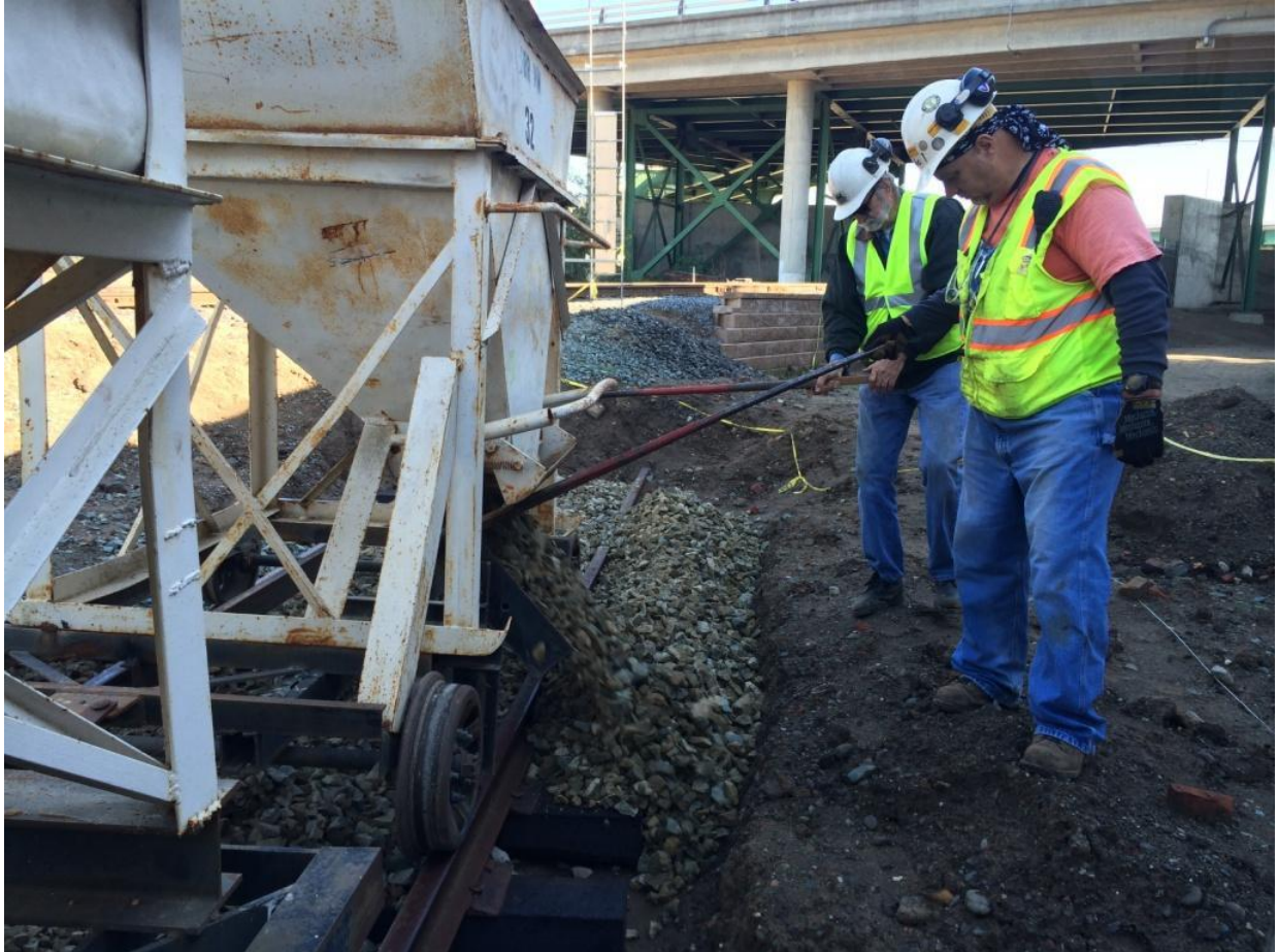
Alan and Mike F. ballast the north end of the Whisker Track
