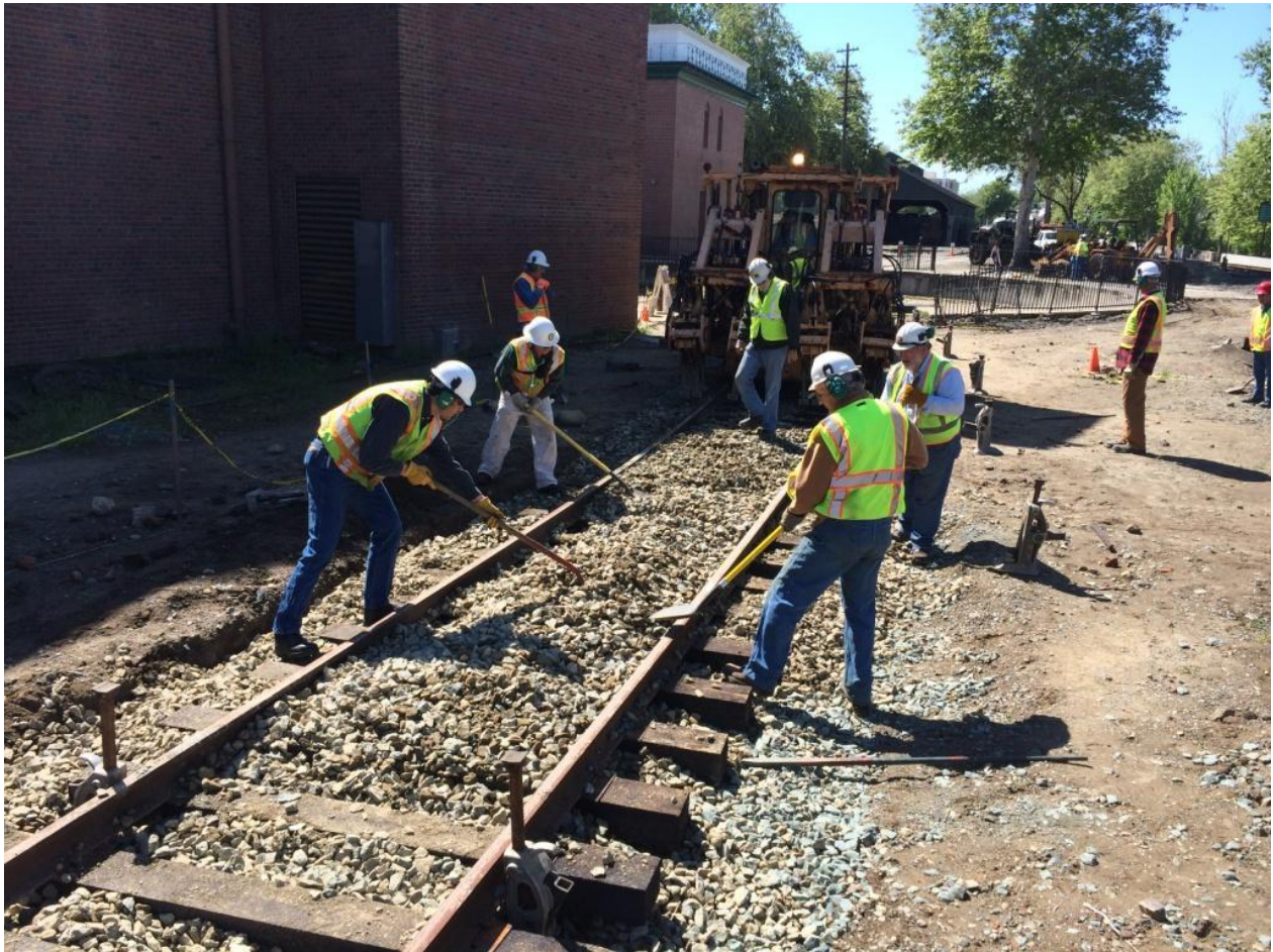
John, Steve, Mike H., and Frank spread ballast in anticipation of the tamper's arrival
