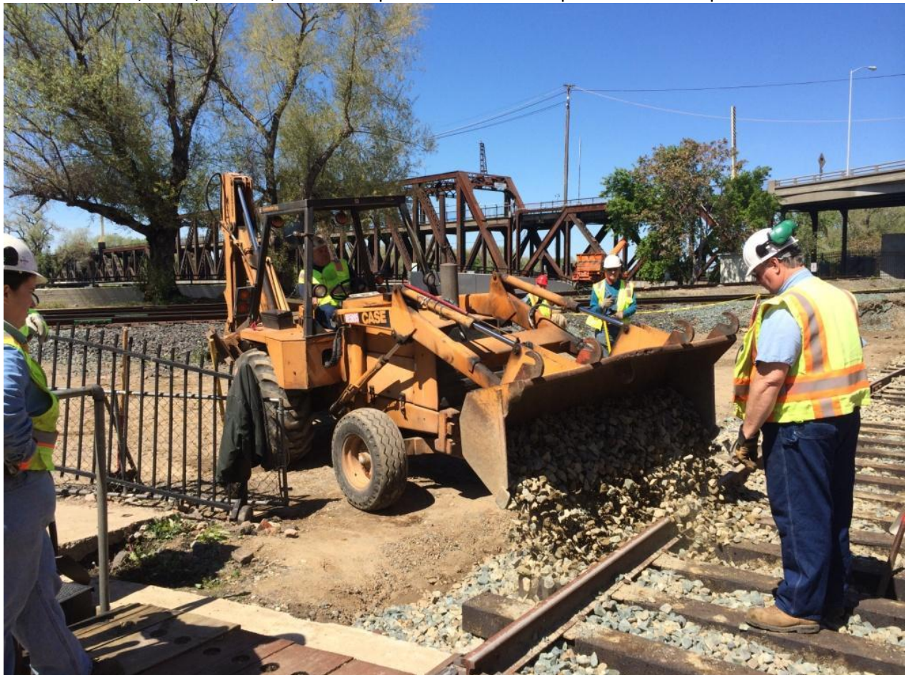
"Hot-rod" Harry V. brings a load of ballast to reinforce the south-west end
